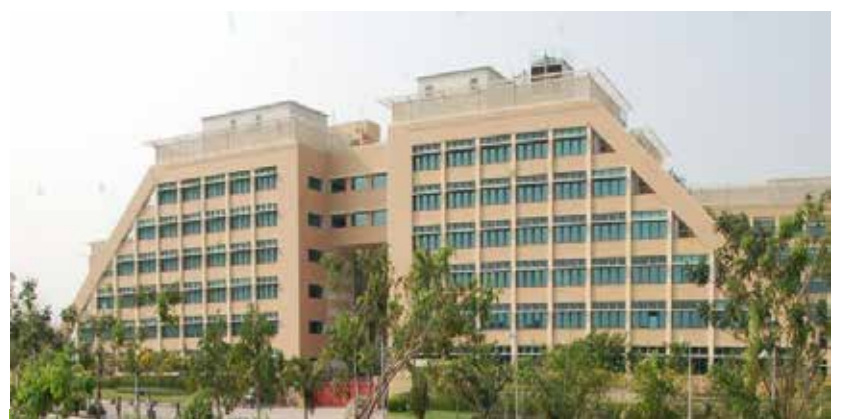
Ultra high efficiency building at Infosys Hyderabad
