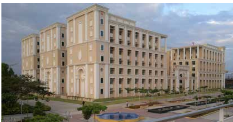
Ultra high efficiency building at Infosys Mysore
